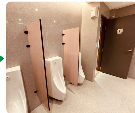
▲ After old stone materials are removed, they are crushed, screened, and re-pressed into recycled quartz stone, which is then re-laid in the original space. Depending on the mix of raw materials, recycled quartz stone can present a variety of textures and offers flexibility for large-area applications, making it suitable for use as a building material.
