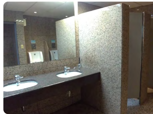
▲ After old stone materials are removed, they are crushed, screened, and re-pressed into recycled quartz stone, which is then re-laid in the original space. Depending on the mix of raw materials, recycled quartz stone can present a variety of textures and offers flexibility for large-area applications, making it suitable for use as a building material.
